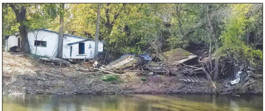
Collapsed Dance Hall, circa September 2021.
