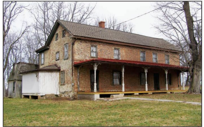
Samuel Painter, Jr. House at Oakland and Harvey Roads.
